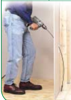
Flexible steel drill bits are perfect for installing wire or cable inside existing walls.
